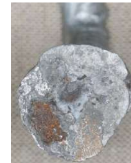
When welding reinforcement bar 11
