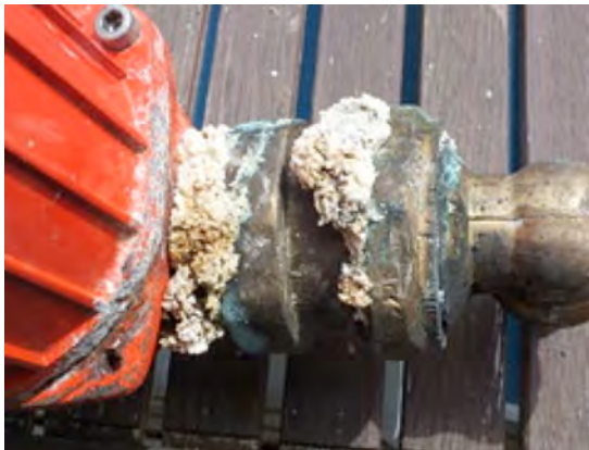
The limescale from seepage at this pipe pump junction proves the water is hard
