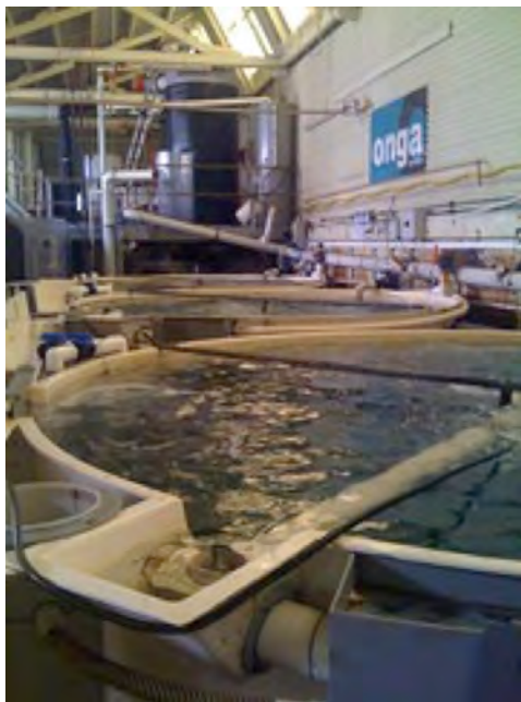
RAS filtration removes organic solids, lowering BOD and strips ammonia
