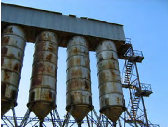
Silage needs to be securely contained to eliminate high BOD discharges
